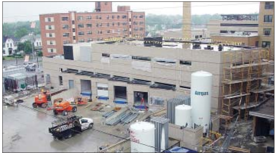
Overhead shot of the Loading Dock prior to opening.
