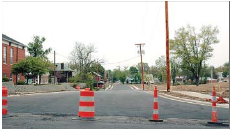
Charles Street after the final paving, before lanes were striped.
