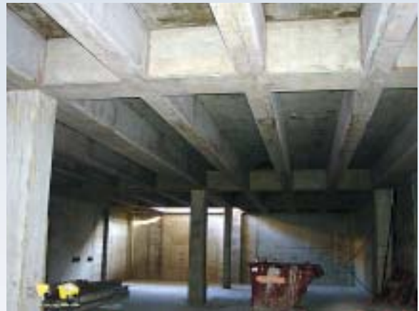
First floor of loading dock after removal of deck formwork.
