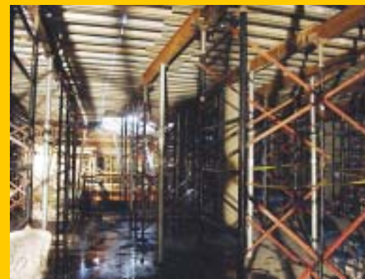
First floor of loading dock...deck shoring for the second floor.
