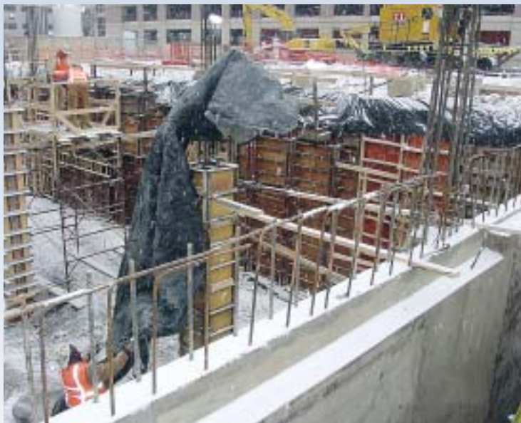
Thermal blankets are applied to newly poured concrete.
